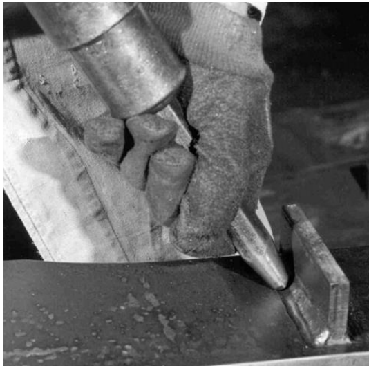
Hammer peening fillet weld toe
