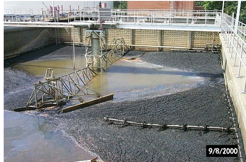
Sludge in the sedimentation basin http://www.norfolk.gov
