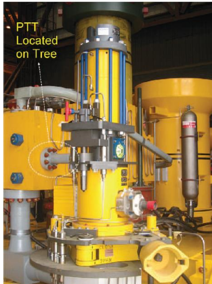
Figure 22-38 PTT Located on a Subsea Xmas Tree
