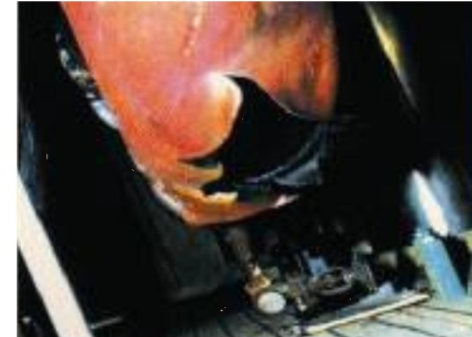
Failure downstream of the LCV in the reheater drain line at Millstone unit 2, 1991.
