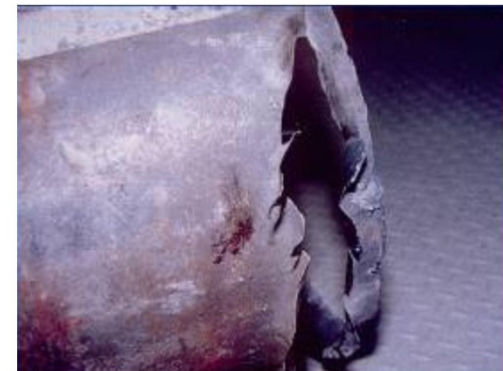
Failure of 14" heater drain extraction line to high pressure heater at Arkansas unit 2, 1986
