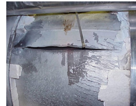
Failure of the Feed-water Heater Point Beach Unit 1, 1999
