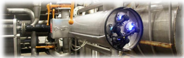
Drinking Water Treatment (UV/H 2 O 2 system)
