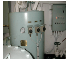
Hot Water Calorifier
