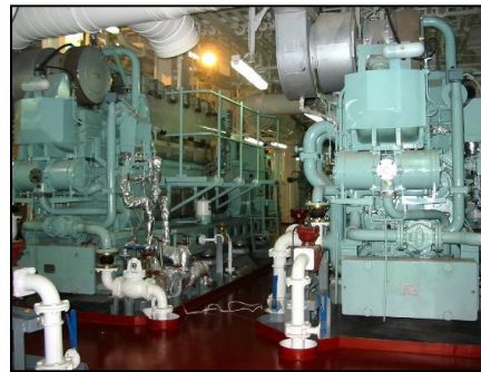
Example of outfitting in engine room
