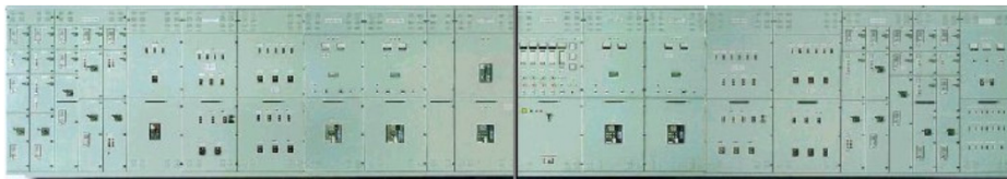
Example of switchboard
