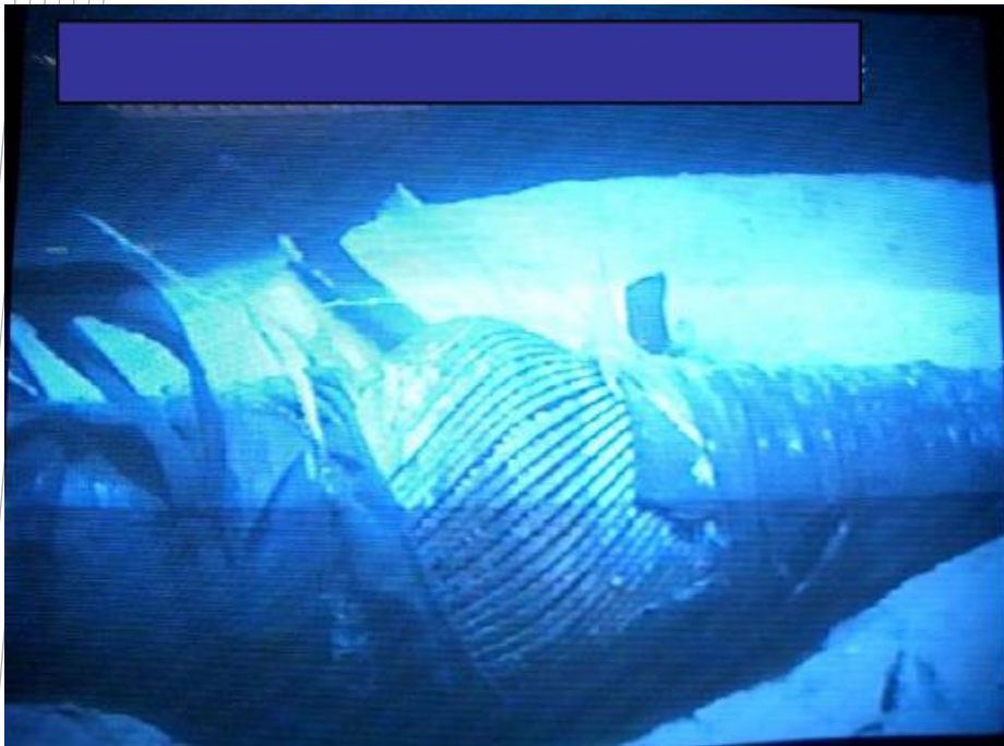
Flowline failure (Operated below min. pressure limit)
