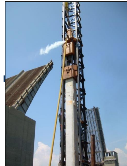
Stream/Air Hammer: Ram lifted by steam or compressed air
