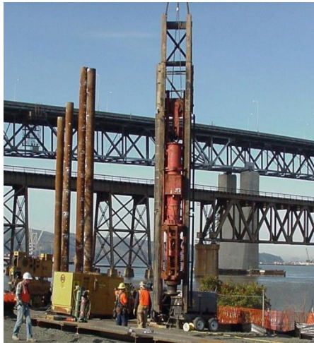
Diesel Hammer: Self-contained driving unit within cylinder
