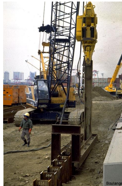
Water Jetting: Water jetting to assist in driving piles by reducing friction and loosening soils with high pressure
