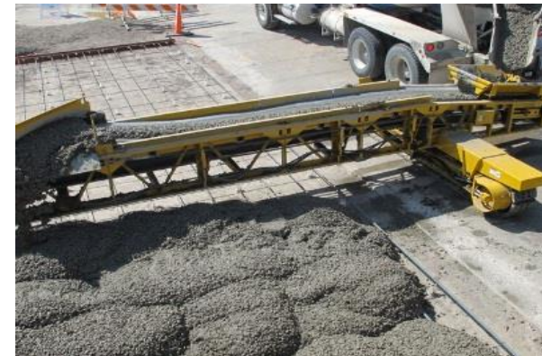
A belt conveyor to place roller-compacted concrete
