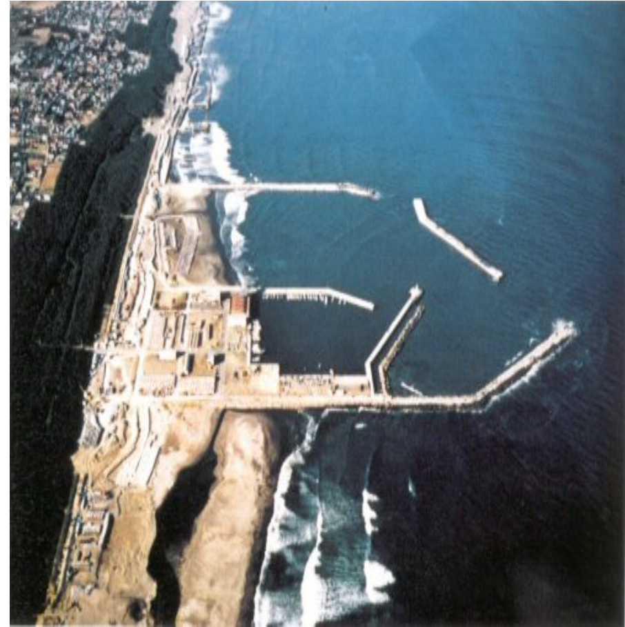
Fig. 1.10 Breakwater for harbors
