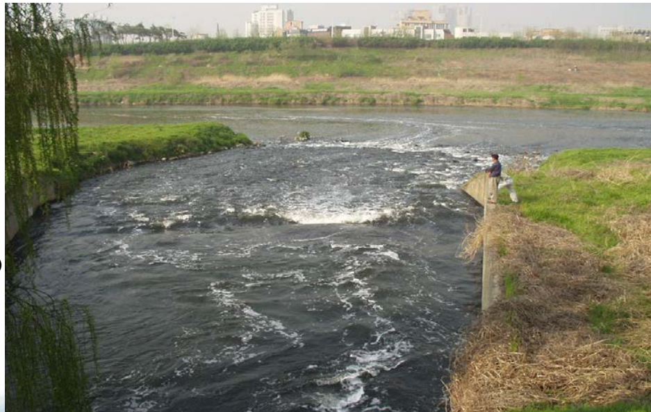
Fig. 1.4 Effluent discharge through open channels (Tancheon STP)
