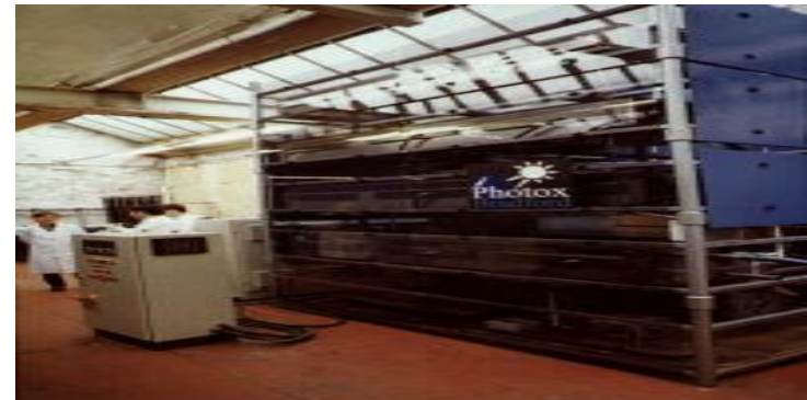
Water purification (Photox Bradford)
