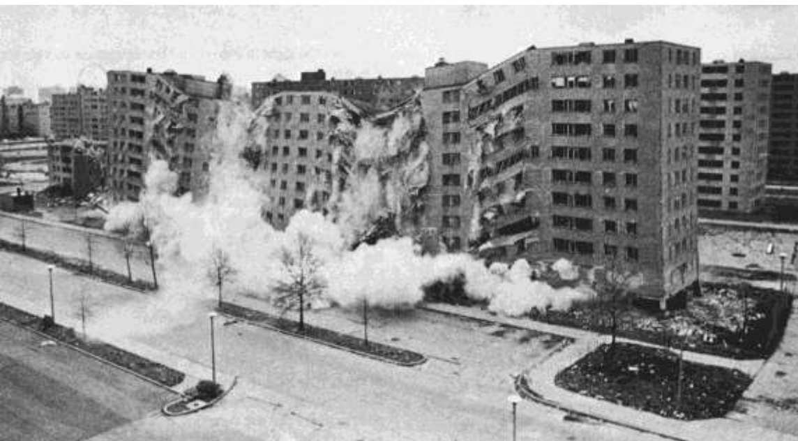
Pruitt Igoe demolition 1971
