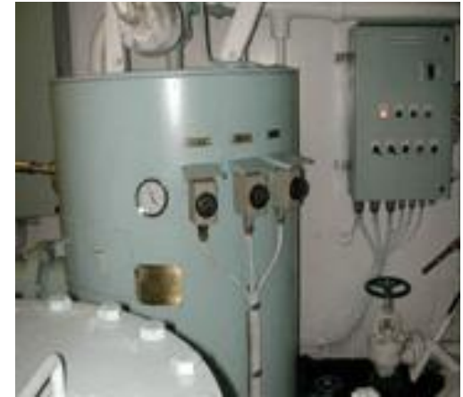
Hot Water Calorifier
