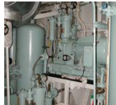
6. Main Air Compressor
