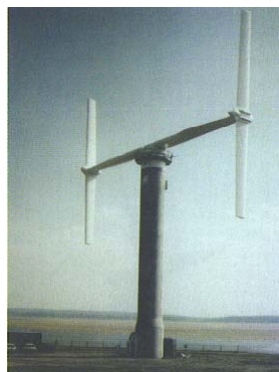
Figure 7.17 500 kW 'H'-type VAWT at Carmarthen Bay, Wales
