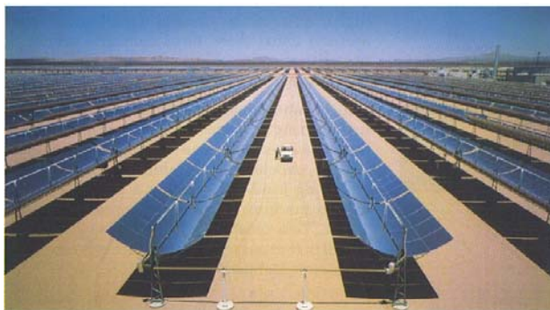
Figure 2.44 SEGS solar collector field at Kramer Junction in southern California
