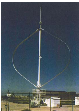
Figure 7.16 Seventeen metre diameter Darrieus-type VAWT at Sandia National Laboratories, New Mexico, US
