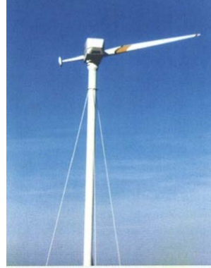
Figure 7.14 A single-bladed horizontal-axis wind turbine (MBB 600 kW)
