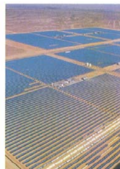
Figure 2.45 SEGS solar collector field – aerial view
