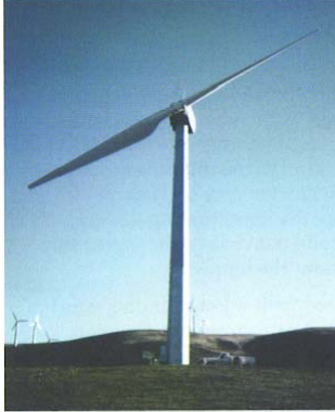
Figure 7.12 A two-bladed horizontal-axis wind turbine (WEG 400 kW)
