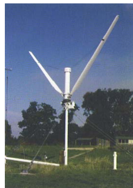
Figure 7.18 'V'-type VAWT prototype at the Open University test site, Milton Keynes
