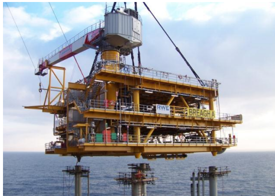
Installation of Breagh Alpha platform (2000 tonnes)
