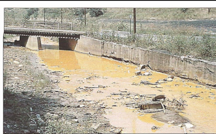
◆ FIGURE 13.23 Rust-red sludge of acid mine drainage from West Virginia coal mines that were abandoned in the 1960s. The acidic water has eaten away at the Portland cement-based concrete retaining wall, and the bridge supports will soon share that fate. Problems such as this are rarely caused by modern surface mines, because current mining and reclamation practices eliminate or minimize acid mine drainage.
