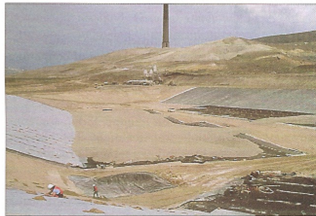
◆ FIGURE 13.35 Preparation of a repository site for contaminated smelter-flue dust near Anaconda, Montana. The pit will have a heavy polyethylene liner.
