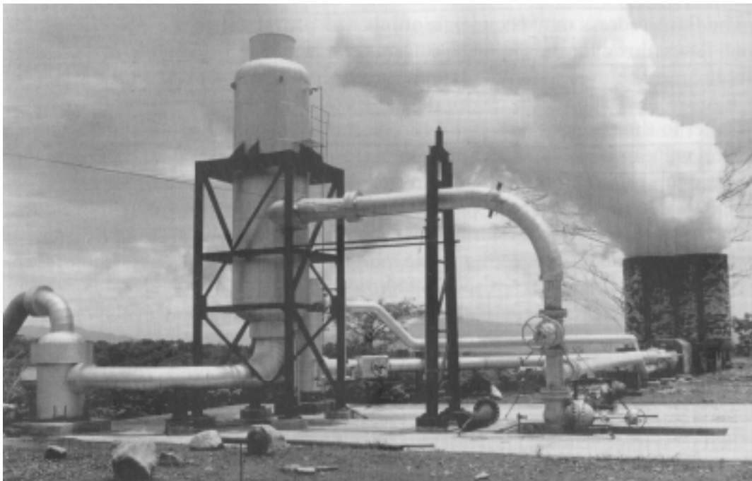
Wellhead separator system at Ahuachapan, El Salvador (DiPippo, 2008)
