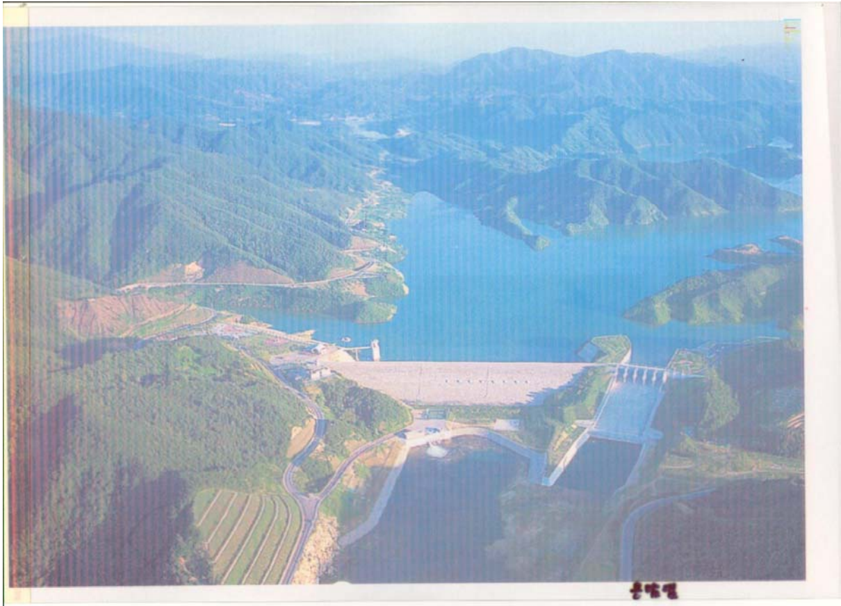
Yongdam Dam at Guem River (Rock Fill Dam)
