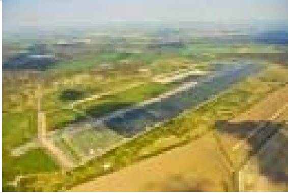
Germany, Brandis (24 MW) (40 MW is planned.)
