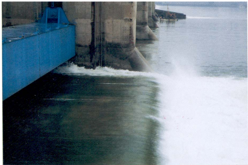
Jamshil submerged weir with gate opened ( Q = 200 \text{ m}^3/\text{s} )
