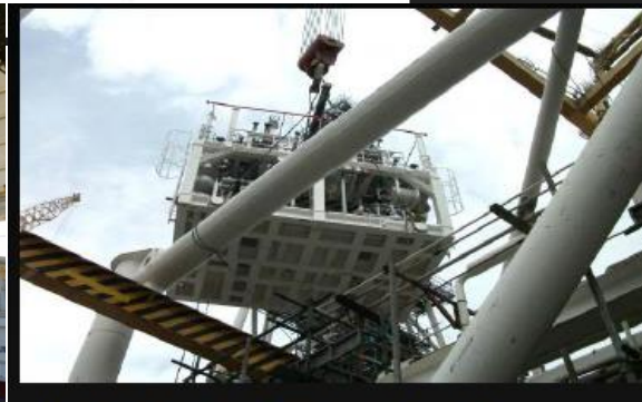
Booster Gas Compressor
