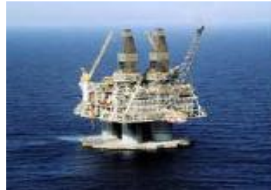
<Exploration and Production of the Natural Gas>
