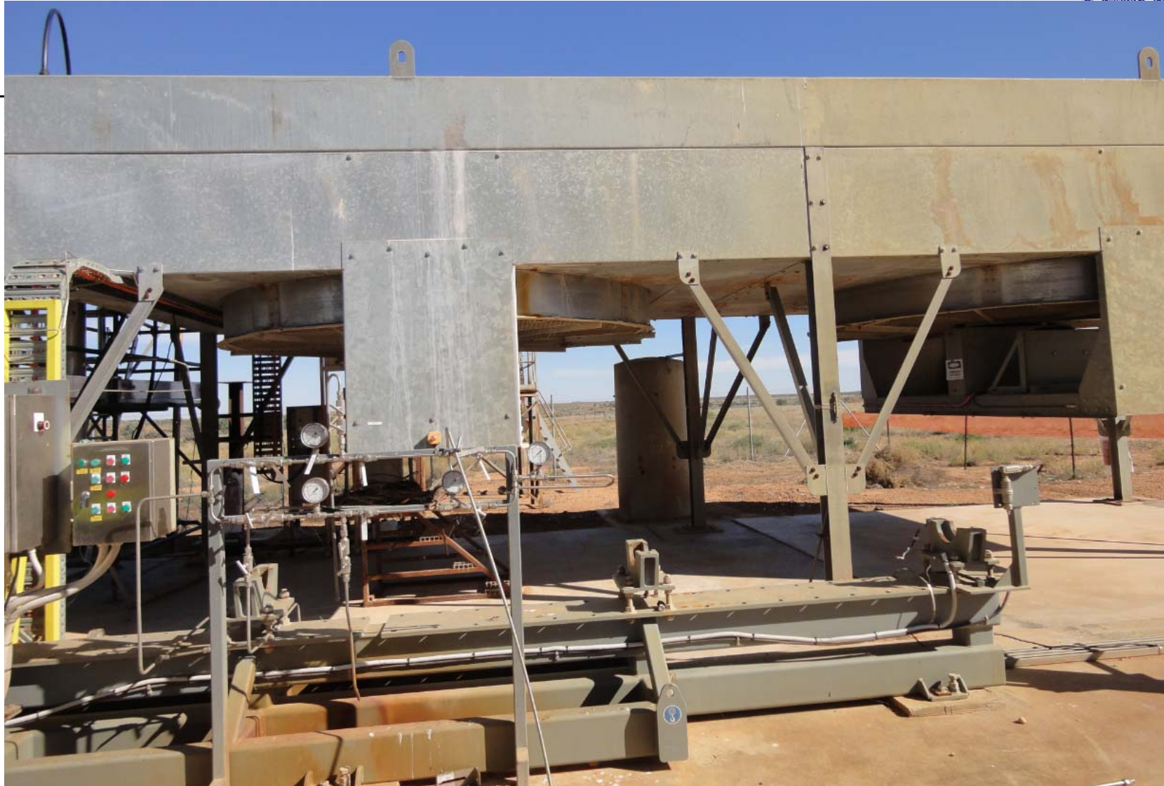
Air cooler and injection pump
