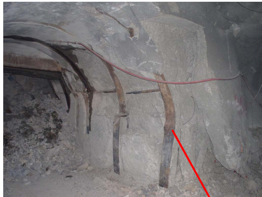
Deflected steel beam
