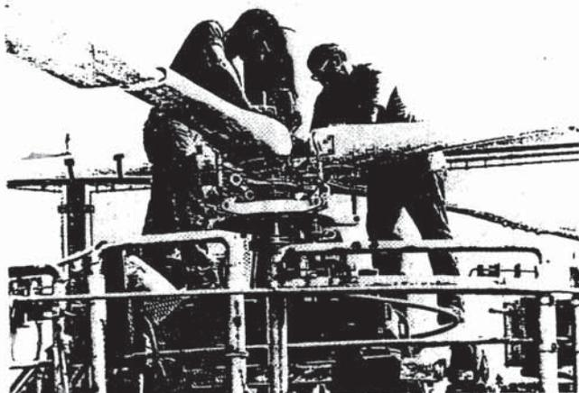
Fig. 16 S-76 BMR demonstrator on whirl tower
