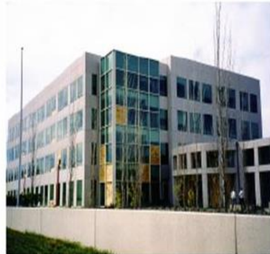
The U.S. Borax Building following the Northridge earthquake
