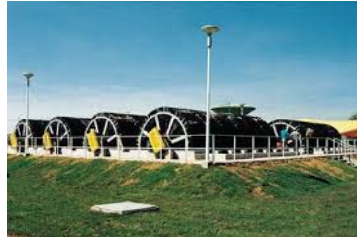
Rotating biological contactor
