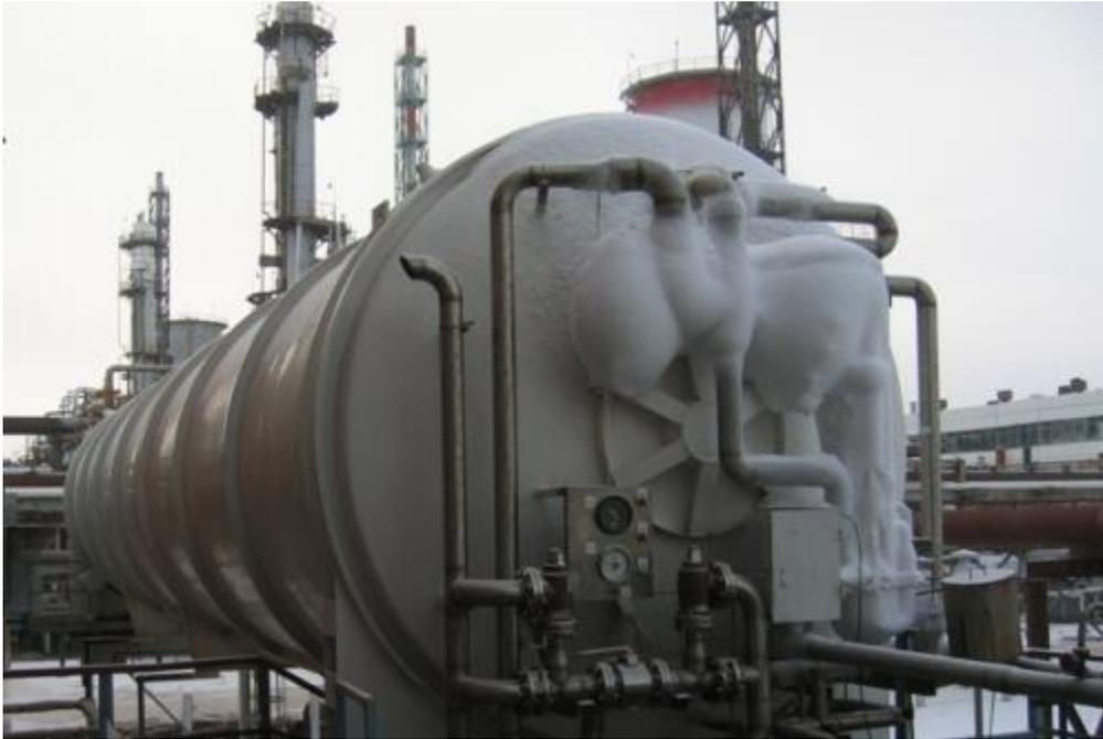
Created by NPO "GELIYMASH", liquefiers of helium with liquid helium capacity of 700 l/h were delivered to the biggest European helium center - Orenburg Gas Processing Plant.
