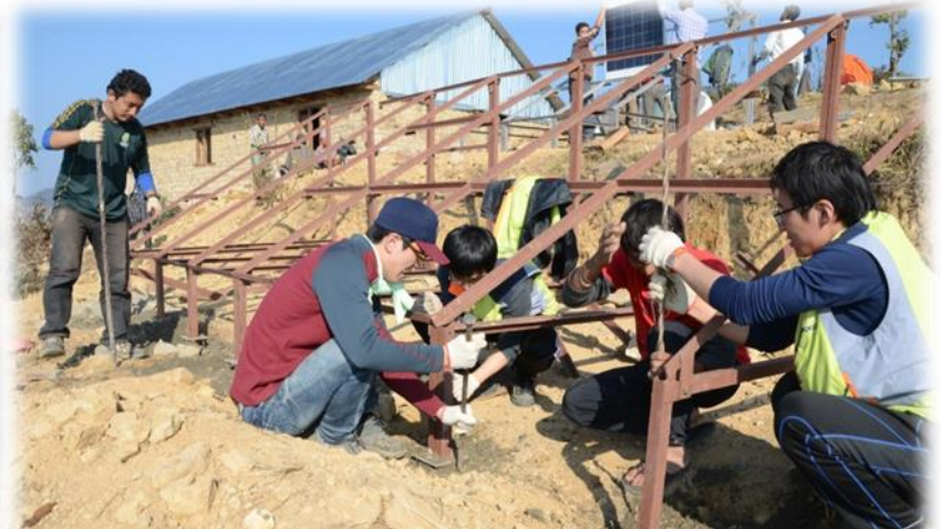
Construction of frames
