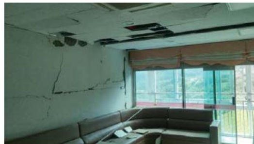
Damage observed in a 3-story RC Building (Ulju, Ulsan)_ ceiling and brick wall failure
