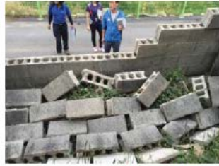
Unreinforced block wall fallen down
