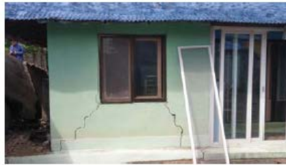
Typical corner cracking at opening
