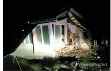
Failure in an already poor (non-engineered) construction
