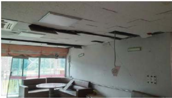
Damage observed in a 3-story RC Building (Ulju, Ulsan)_ ceiling and brick wall failure
