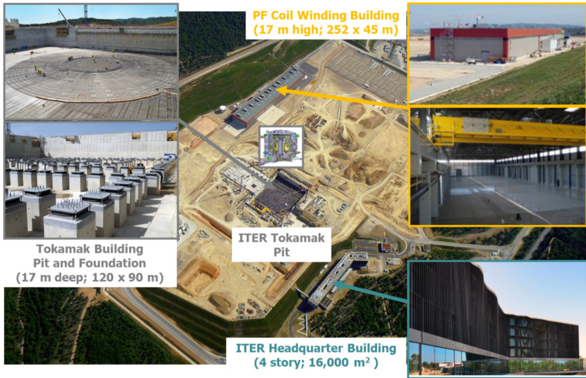
Figure 2. Recent views from the ITER construction site, near Saint-Paul-Lez-Durance, France.
