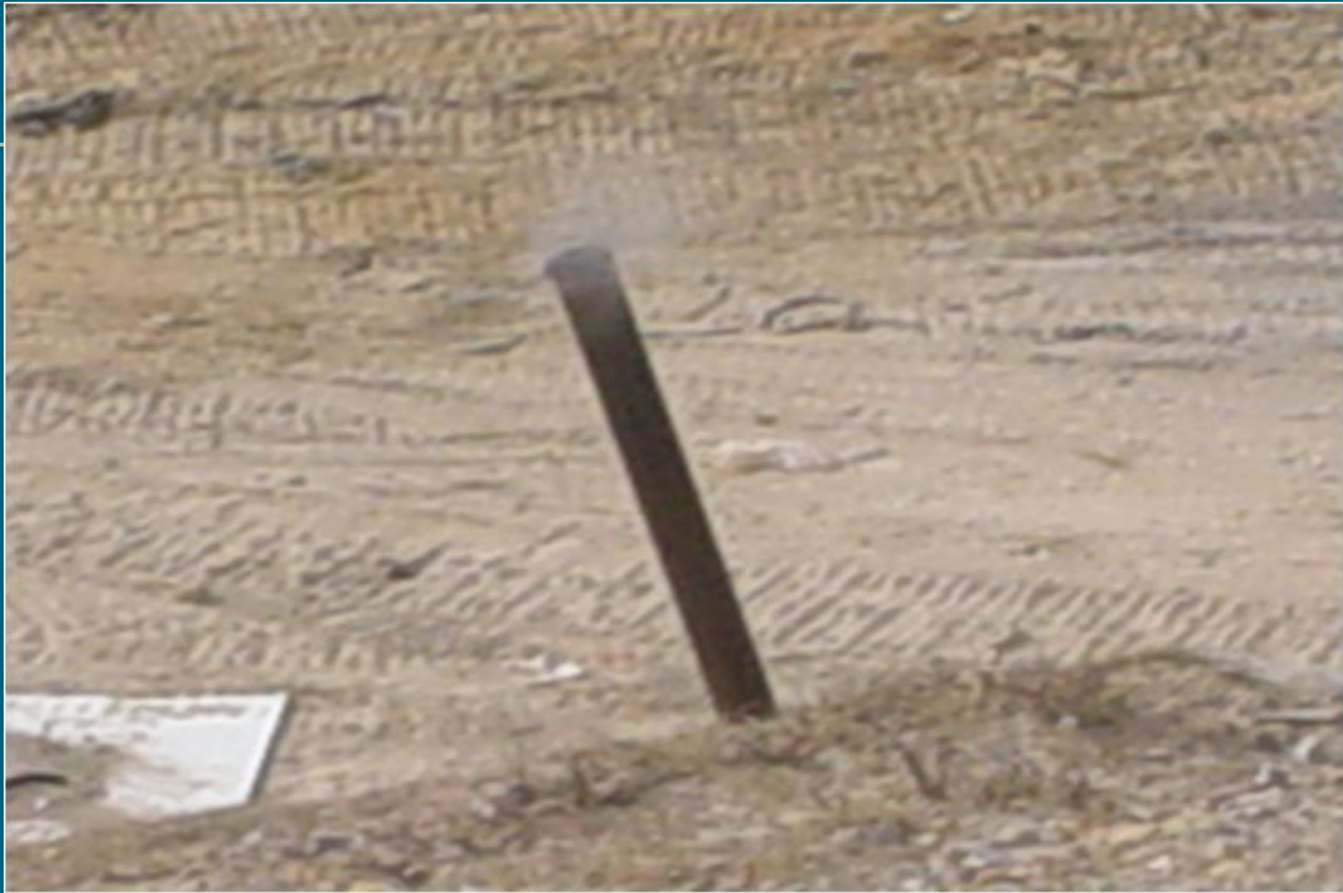
Landfill gas released through the gas vent
