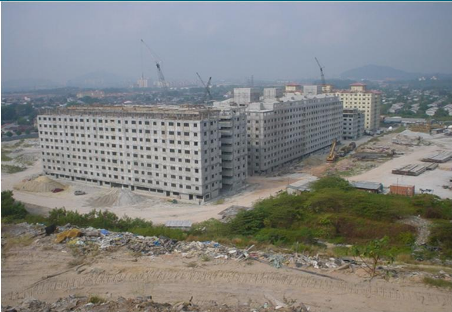
Construction of low cost apartment near landfill site
