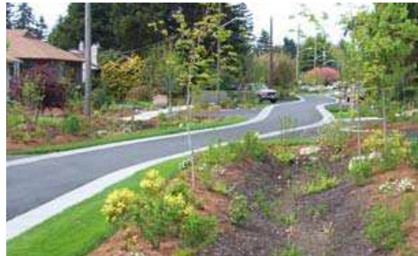
An LID project in Seattle, USA ( http://www.mapc.org )
