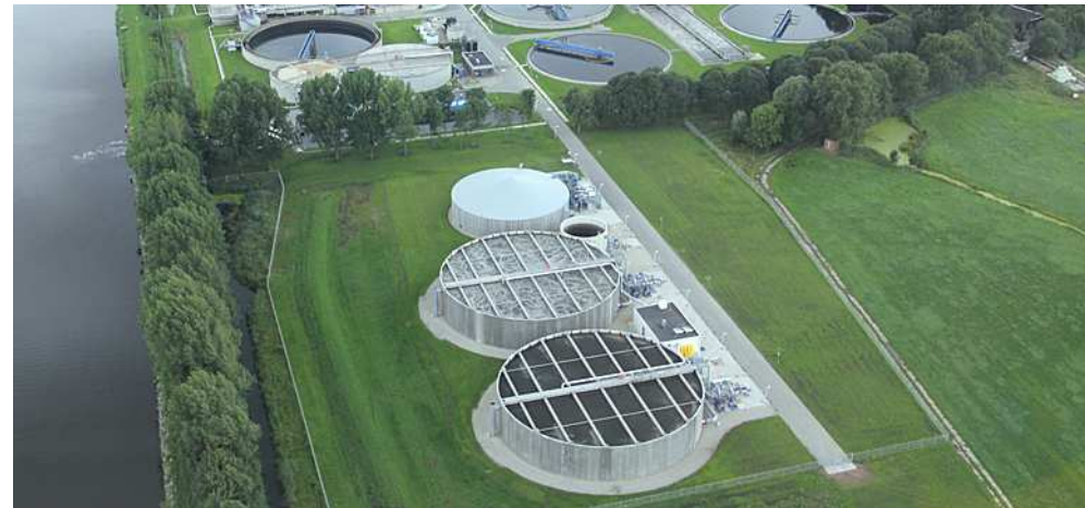
WWTP in Garmerwolde, the Netherlands (2010~)
