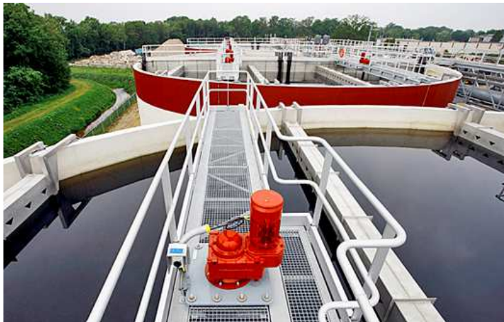
WWTP in Epe, the Netherlands (2010~)
