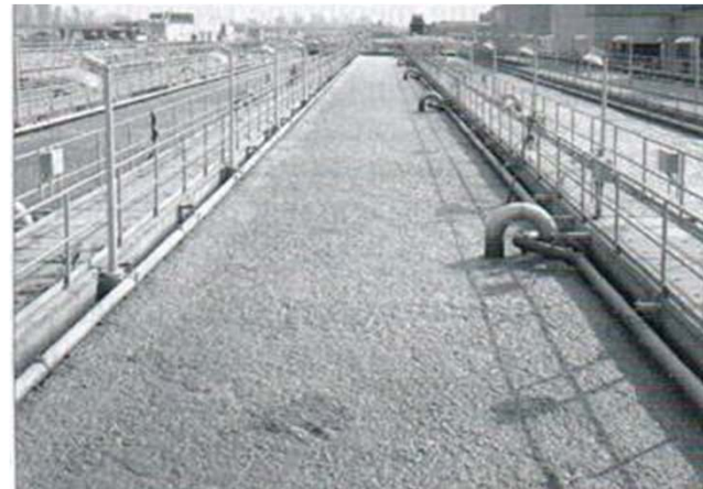
Foam caused by Gordonia amarae accumulated on the surface of an aeration tank
