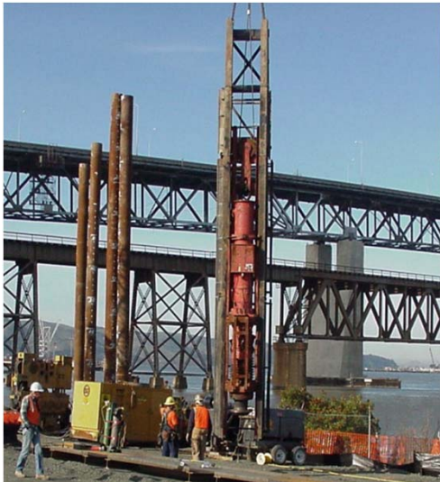
Diesel Hammer: Self-contained driving unit within cylinder
