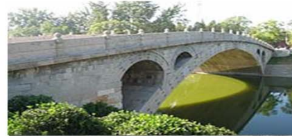
Great Stone Bridge in China
