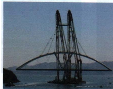
(a) Floating crane 예항
