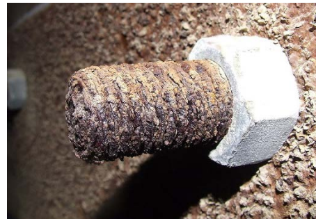
Corrosion on exposed metal bolt
