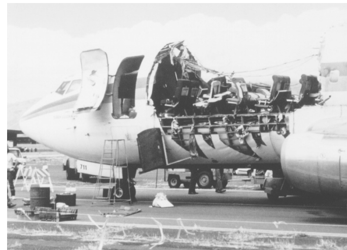
Figure 1.11 Fuselage failure in a passenger jet that occurred in 1988.
