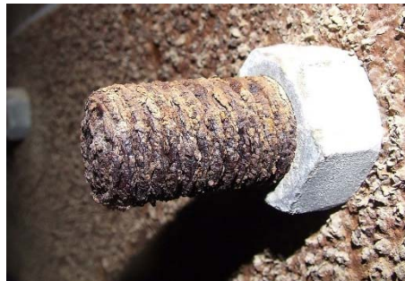
Corrosion on exposed metal bolt
