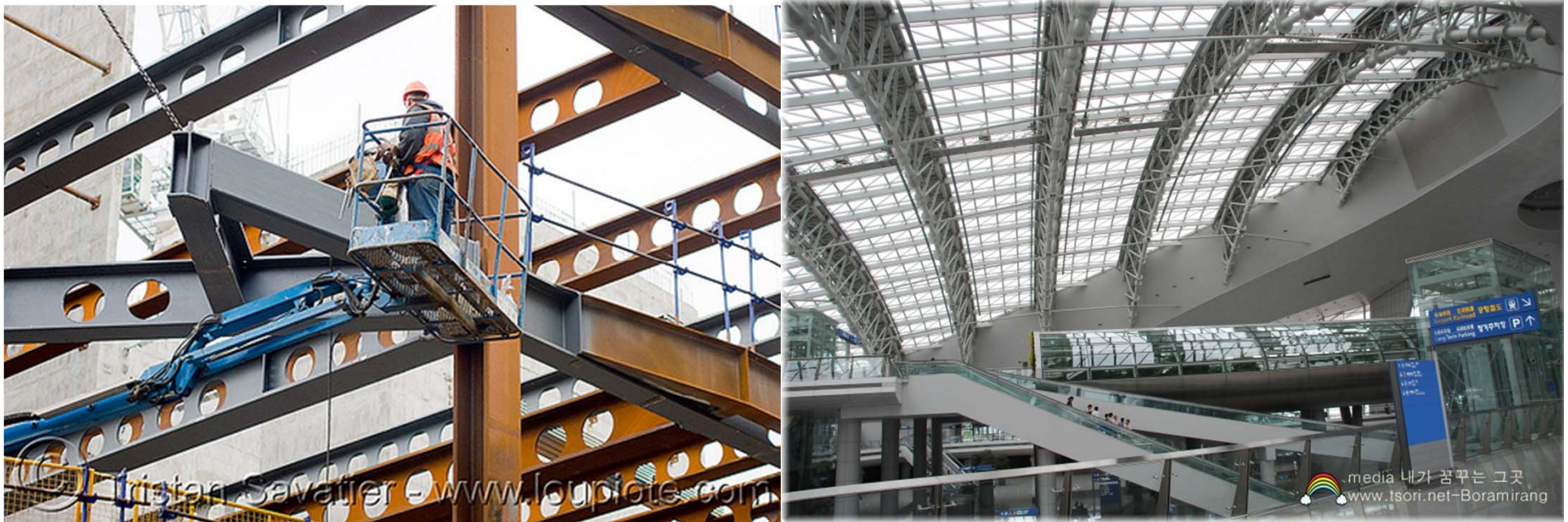
Steel frame of building
