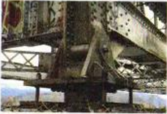
Pin support on old truss bridge (© Barry Goodno)
