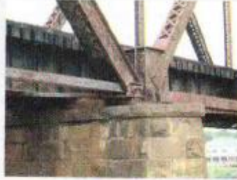
Bridge with pin support (Courtesy of Joel Kerkhoff, P.Eng.)
