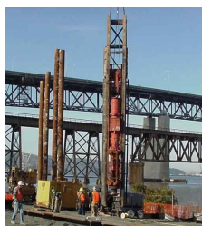
Diesel Hammer: Self-contained driving unit within cylinder
