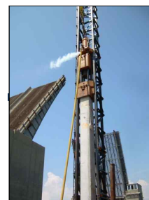
Stream/Air Hammer: Ram lifted by steam or compressed air
