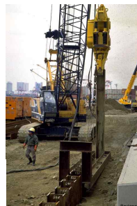
Drop Hammer: Lifted by a hoist line
