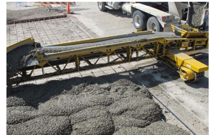
A belt conveyor to place roller-compacted concrete
