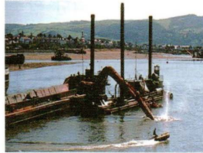
(b) Trench 굴착
