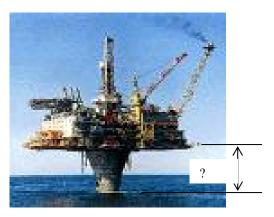
(2) If this ocean is represented by 4.0m significant wave height and 10sec modal wave period, find the wave height of 100-year return period, which waves cannot reach to the deck. (This is an example of short-term prediction.)
