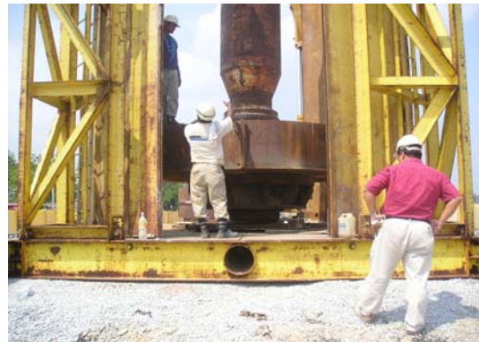
Figure 10: Installation of weight
