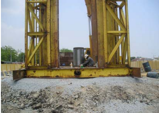
Figure 1. Installation of piston and oil application
