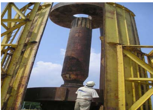
Figure 11: Installation of weight
