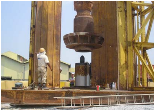
Figure 9: Installation of cylinder
