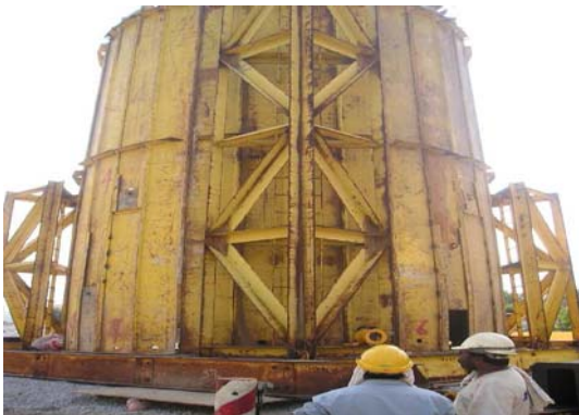
Figure 15. Closing of the structure panels and installation of gravel
