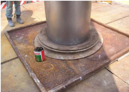
Figure 7: Installation of base plate
