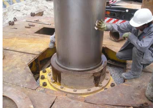
Figure 2. Piston and oil installation
