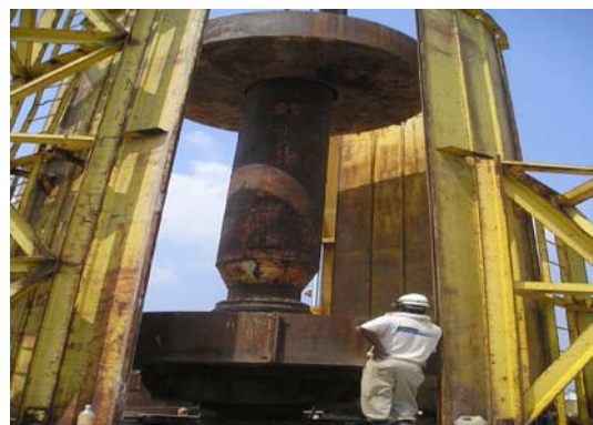
Figure 12: Installation of weight
