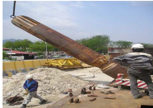
Figure 8: Installation of cylinder
