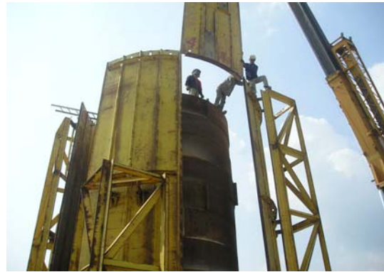
Figure 14. Placing the gravel structure non-supporting panels
