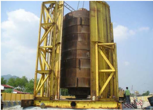
Figure 13. After installation of weight mass
