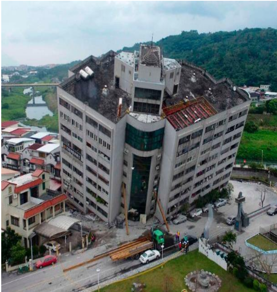
Hualien Earthquake (Mw = 6.4), Taiwan, 2018-02-04
