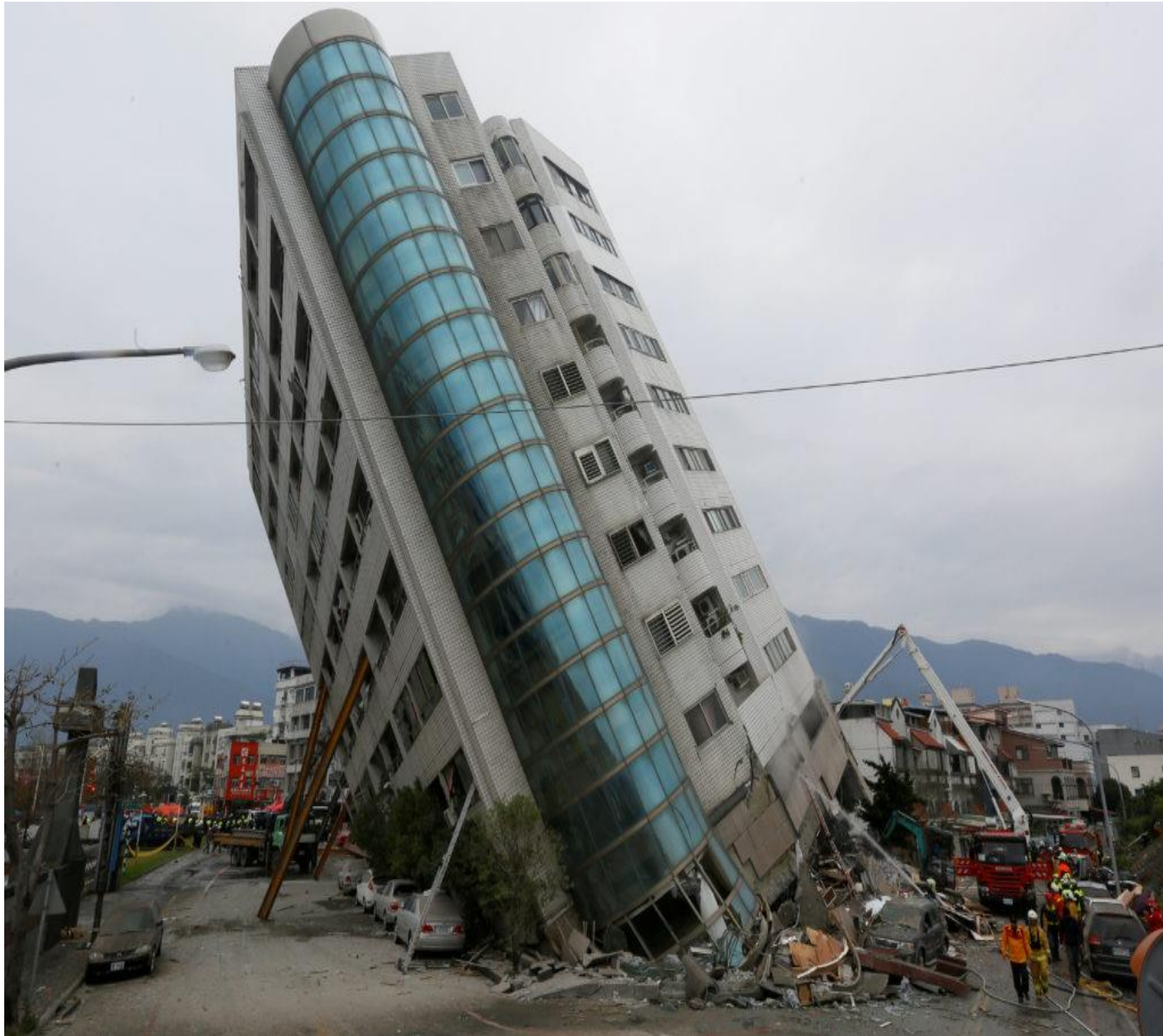
Hualien Earthquake (Mw = 6.4), Taiwan, 2018-02-04
