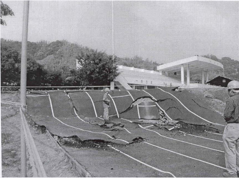
Figure. 1-20 Ground uplift along the fault in the 1999 Chi-Chi Earthquake (Photo by Dr. Farzad Naeim).
