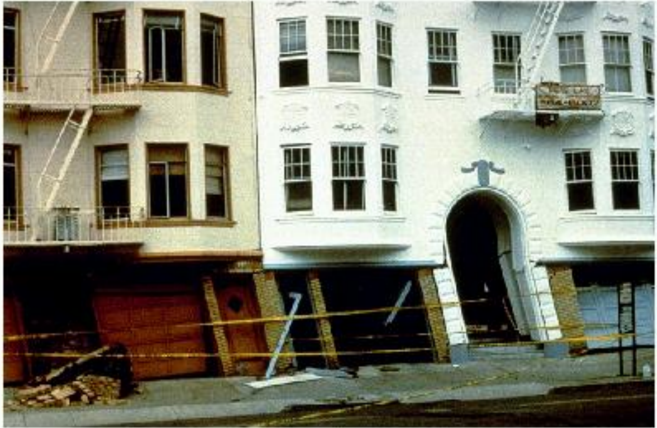
Slides 32 to 35: 'Soft-Story' Building Deformation
