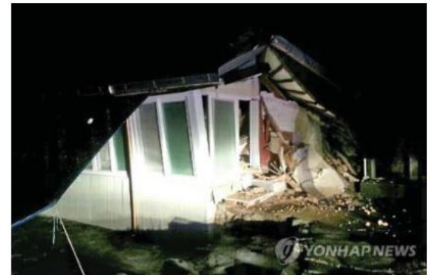
Failure in an already poor (non-engineered) construction
