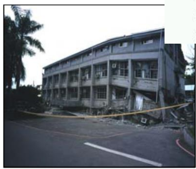
Fig. 7. Elevation of base floor, removal of partition wall, illegal penthouses on roof
