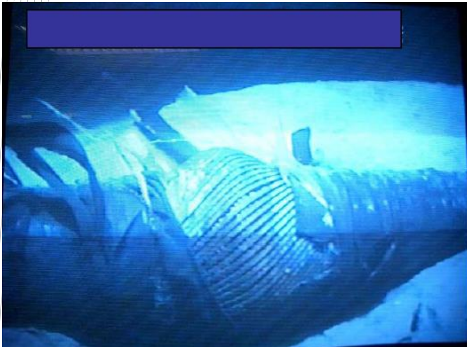
Flowline failure (Operated below min. pressure limit)
