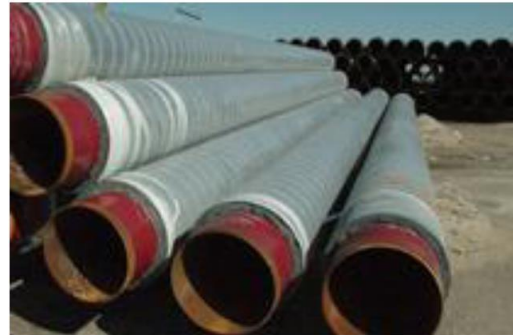
Concrete coated pipeline
