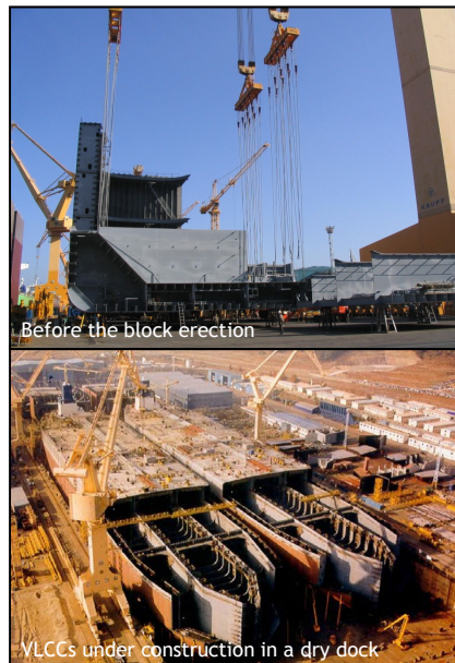
VLCCs under construction in a dry dock
